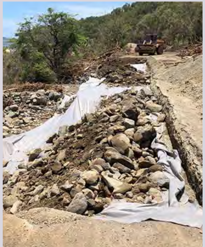
Image: Captain Cook Highway (Cairns–Mossman) emergency works
