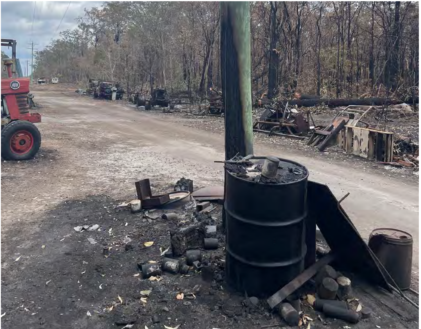
Image: Bundaberg bushfire damage (courtesy: QRA)
