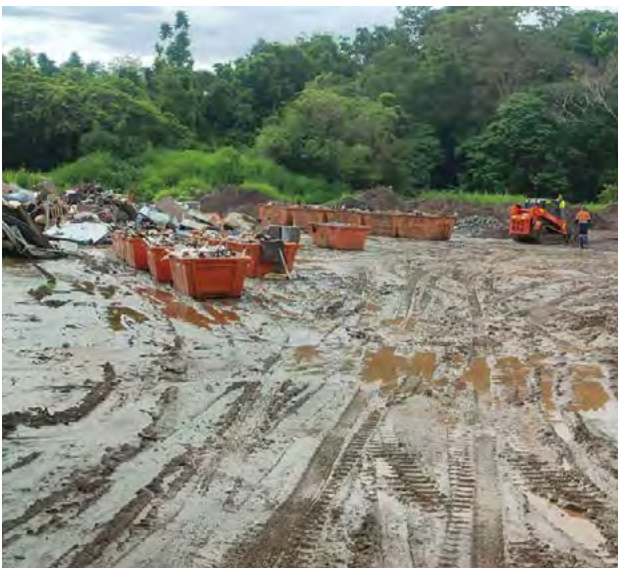
Image: China Creek Road waste staging area with skip bins (courtesy: Department of Environment, Science and Innovation)
