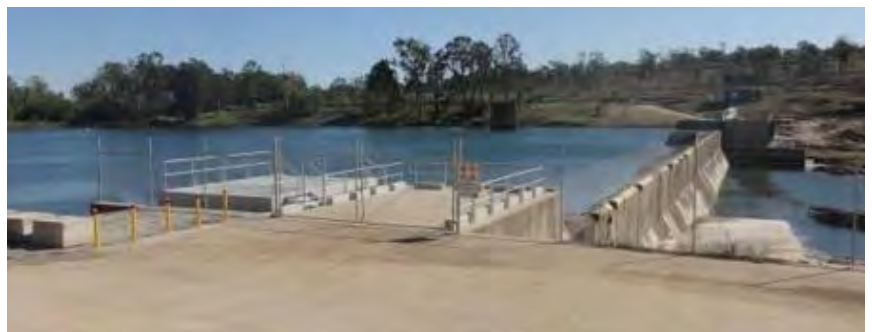
Image: Completed works on the Gayndah Water Supply Intake Station (courtesy: QRA)
