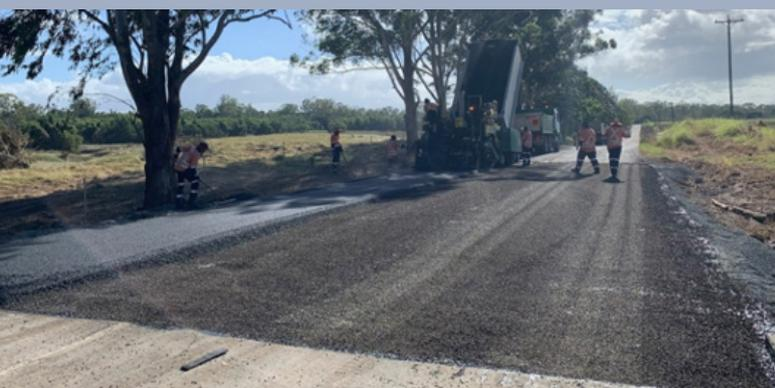
*Image: (top): Mungar Road – pavement damage to culvert west of Mary River Bridge. (Bottom): Mungar Road – emergency pavement repairs to culvert west of Mary River Bridge.*
