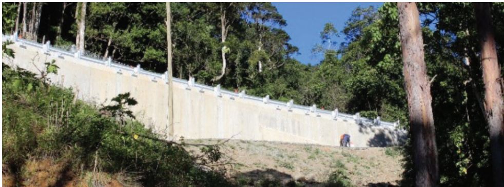
Nerang-Murwillumbah Road – completed works
