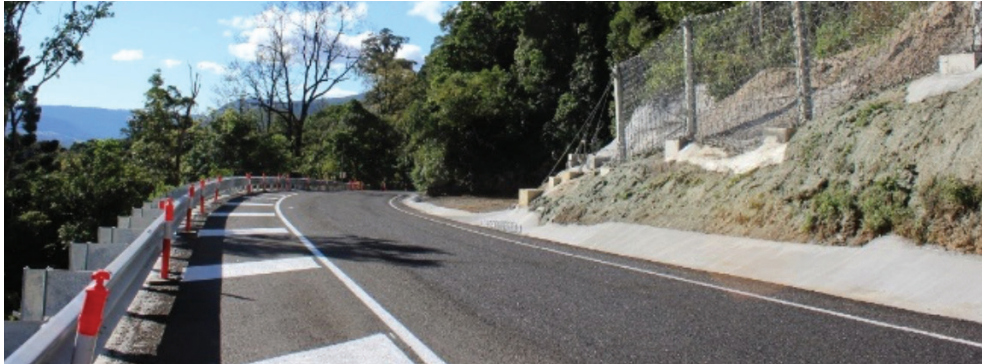
Nerang-Murwillumbah Road – completed works
