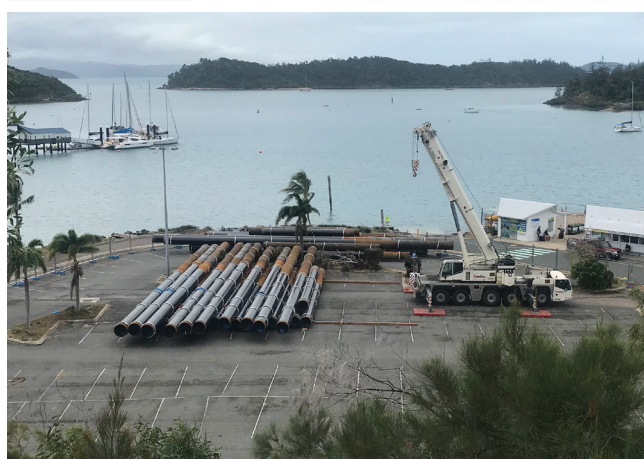
Pile delivery for Shute Harbour, Whitsunday Regional Council
