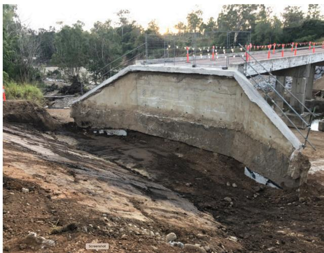
*Alice River Bridge – removal of damaged concrete margins and approach slab*
