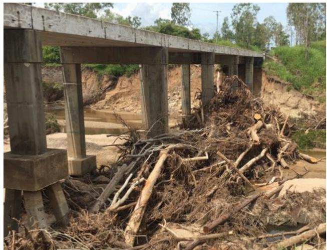
*Alice River Bridge – large debris had to be removed once floodwaters subsided to allow inspection of the bridge piers*
