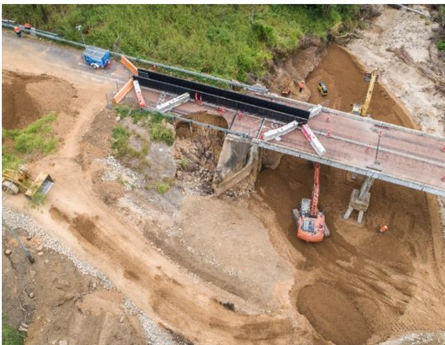
*Alice River Bridge – during works, showing the large void under the western abutment due to scouring*
