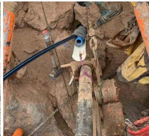
Rock nailing process – white cradle half pipe and blue anchor with grout tubes
