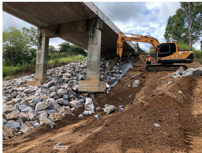
*Alice River Bridge – placing rock protection on the eastern abutment*
