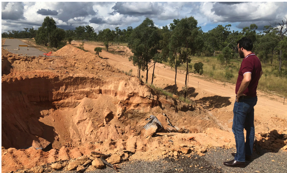
QRA RLO inspecting damage to Laroona Road in Charters Towers
