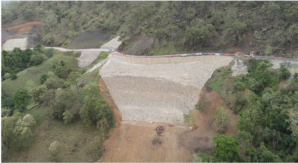
Marlborough-Sarina Road – completed repairs at main slip site
