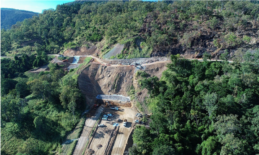
Marlborough-Sarina Road – repairs in progress at main slip site
