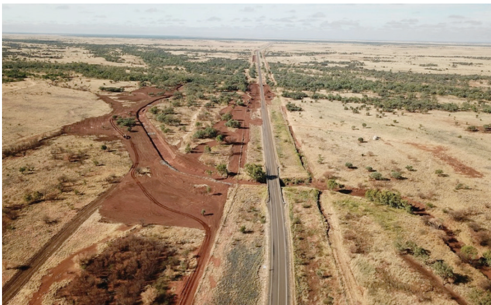
Aerial view of Canal Creek project
