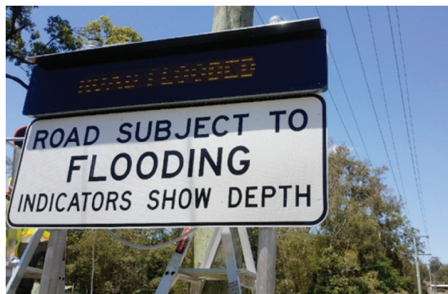
Flooded road smart warning signs
