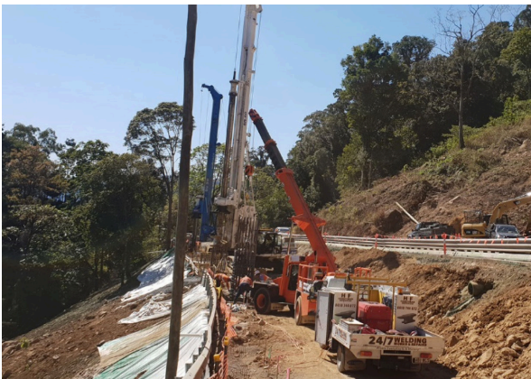
Plant transported successfully following bridge propping measures
