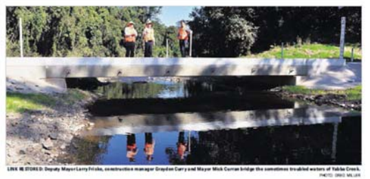
LINA REID FOR D: Deputy Mayor Larry Frislie, construction manager Grayden Curry and Mayor Mick Curran bridge the sometimes troubled waters of Yabba Creek. PHOTO: 2015 WJLW
