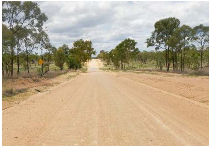
Kennedy Developmental Road— following completion of reconstruction works following 2014 event damage
