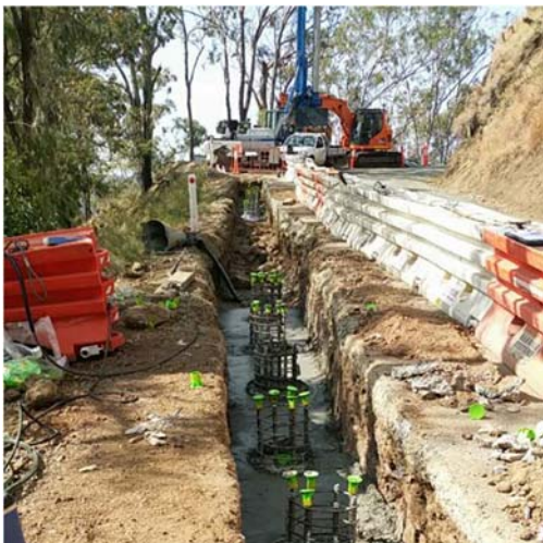
Above: Laying pile foundations at Lamington National Park Road
