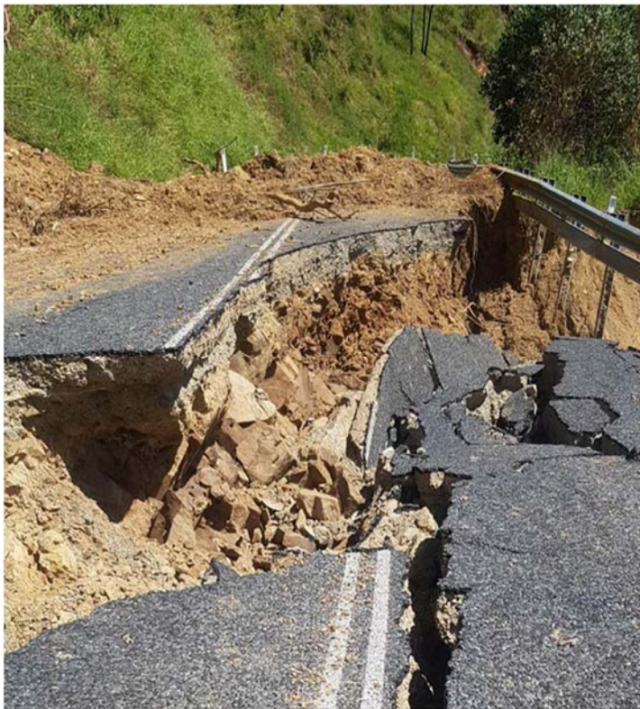
Damage at main slip site on Marlborough–Sarina Road (above), aerial survey showing second major slip profile (above right) and preliminary upslope works at the secondary slip site (right)
