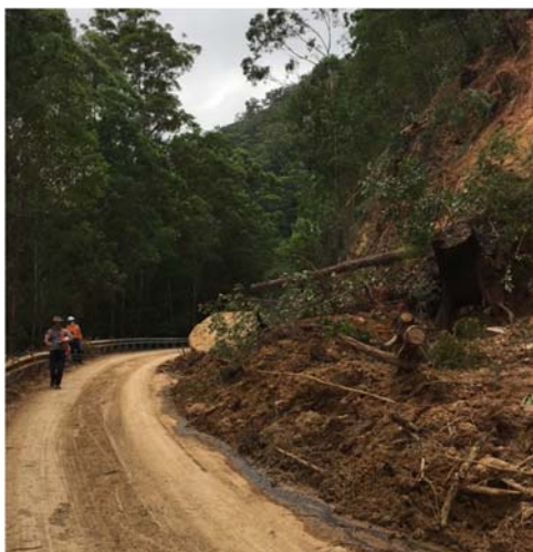
Above: Emergent works on Gold Coast-Springbrook Road
