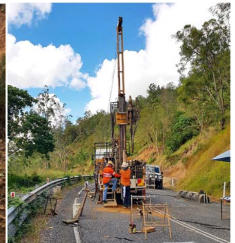
Above: Geotechnical assessment being carried out on Sarina Range
