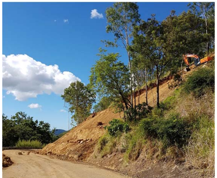
Damage at main slip site on Marlborough–Sarina Road (above), aerial survey showing second major slip profile (above right) and preliminary upslope works at the secondary slip site (right)
