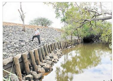
LEVEE INSPECTION: Bundaberg Regional Council Project Manager Warren Paulger examines the finished stabilisation work on the levee bank backing on to Bundaberg Creek at Kendall Flat. The area was significantly eroded in the past two flood events. PHOTO: CONTRIBUTED
