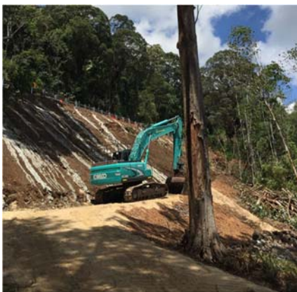
Above: Repairs in progress at Tomewin Mountain Road
