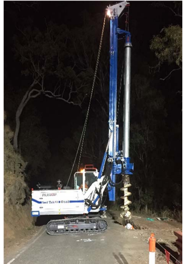
Night works on Lamington National Park Road (above)
