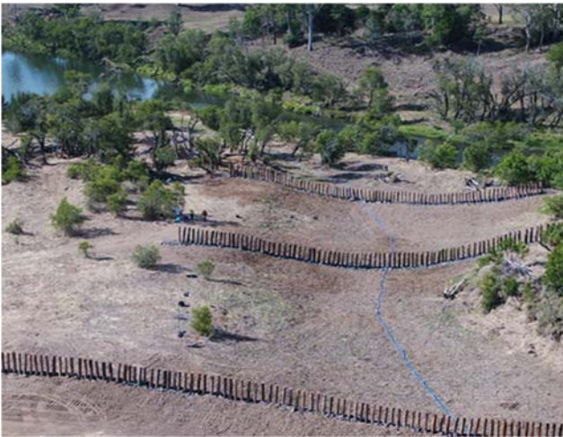
Aerial photo of the pile fields which will provide scour protection in the long term.
