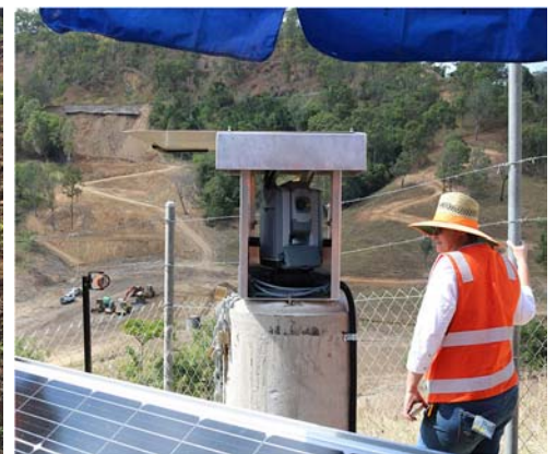
Above: Monitoring station to detect movement at main landslide site on Sarina Range
