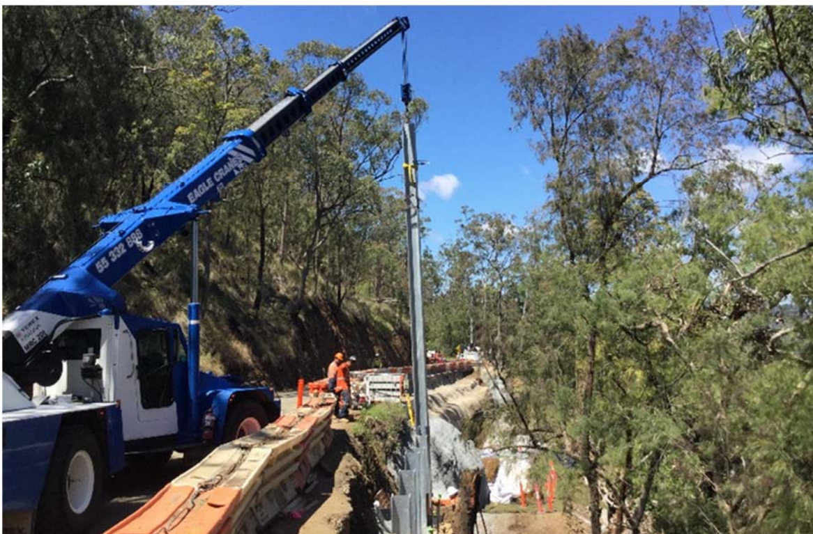
Repairs in progress on Lamington National Park Road (left)
