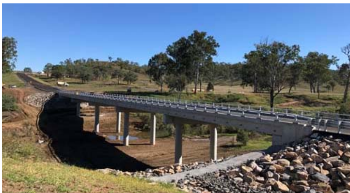
(Above) Burnett River Bridge complete
