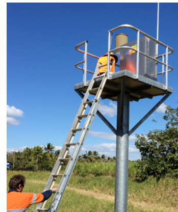
A flood gauge in Burdekin Shire Council
