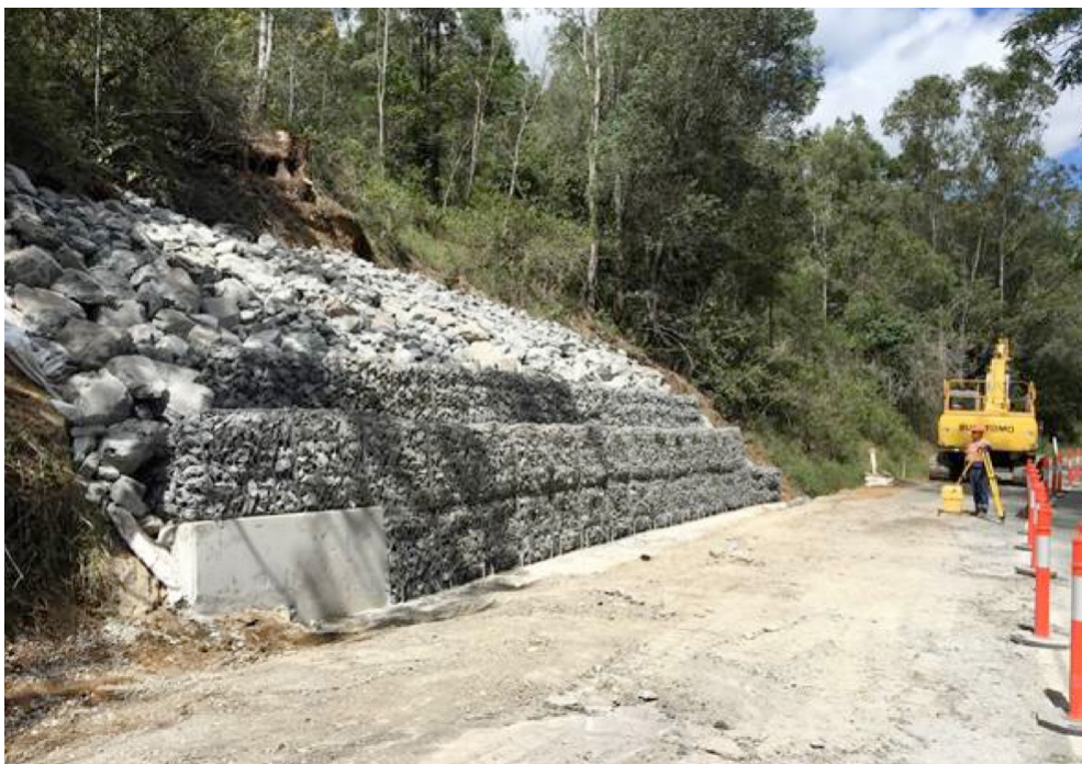
Lamington National Park Road – work complete at Site 64 (Chainage 3)
