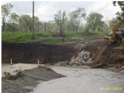
George Bell Crossing washed away in 2013 flood event
