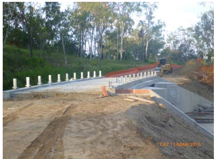
Upper Ulam Road floodway under construction survives Cyclone Marcia - March 2015
