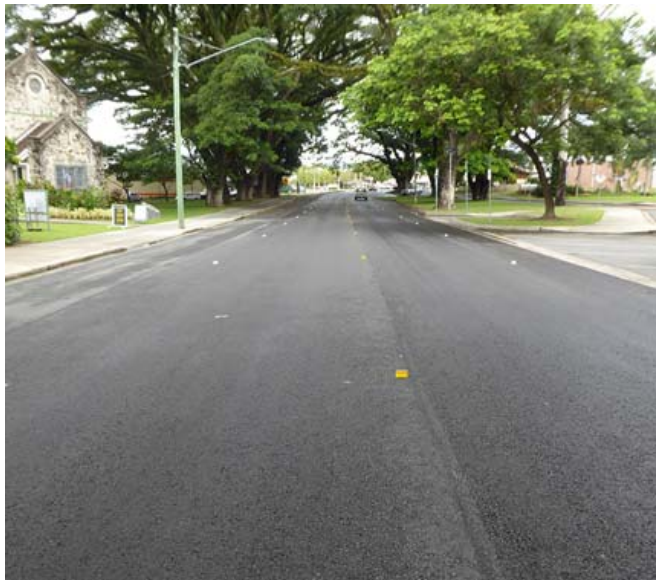
Completed pavement rehabilitation on Mossman–Daintree Road prior to linemarking
