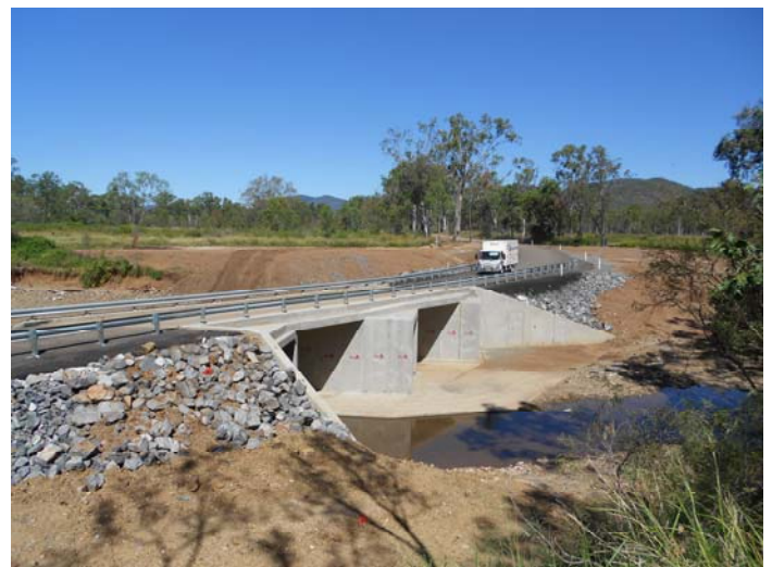
Betterment works complete and in use on Upper Ulam Road.
