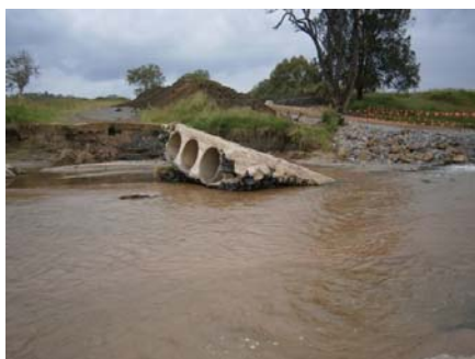
Damage to Ted Skinner Crossing on Esk-Crows Nest Road following 2013 flood
