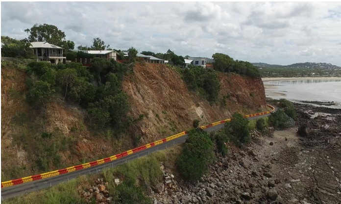
Betterment works will strengthen the upslope and prevent future landslips
