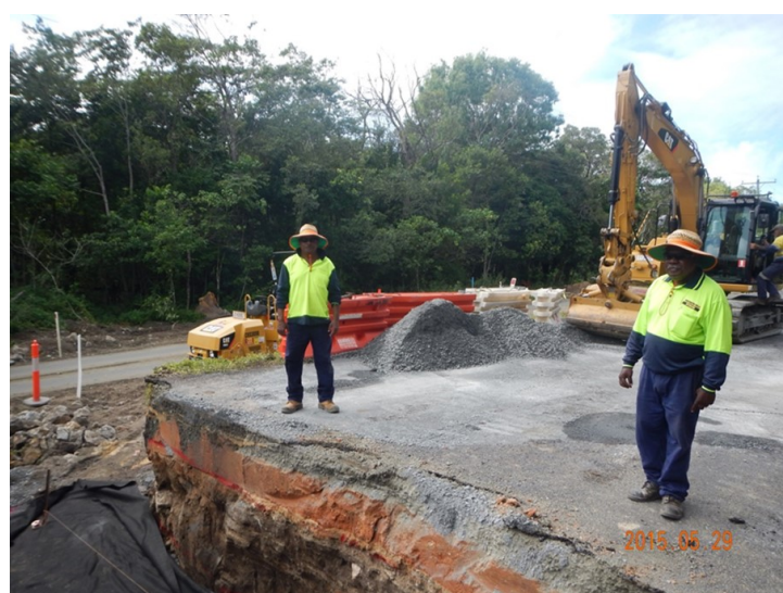
Disaster recovery work underway at Yarrabah
