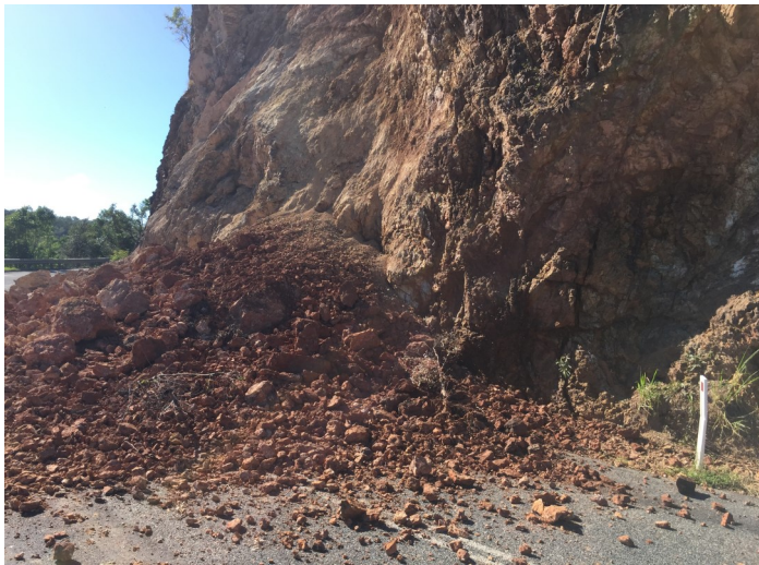
Landslips over the Scenic Highway following Cyclone Marcia – February 2015
