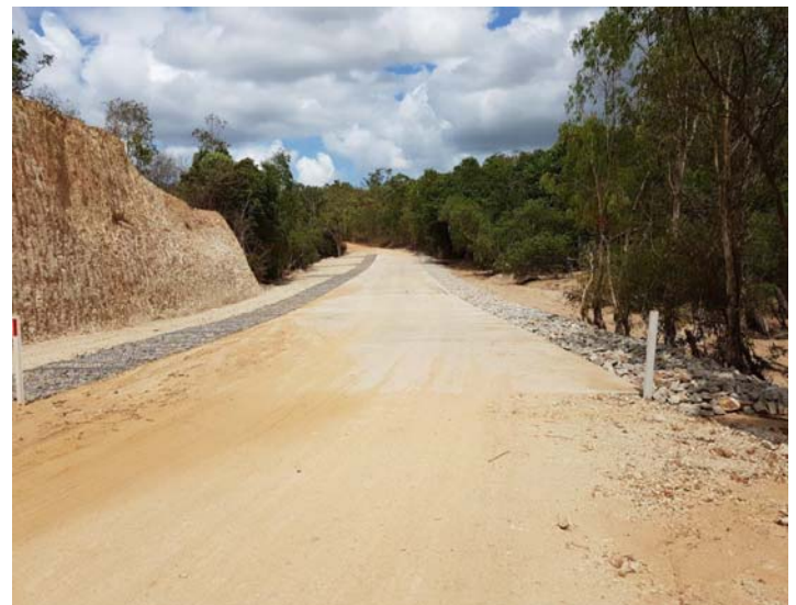
Completed works – 21 December 2016
