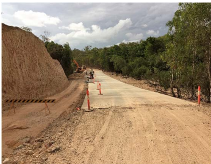
During works - November 2016
