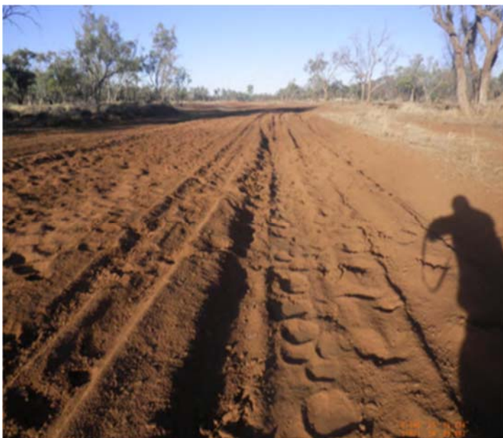
Damage (left), and following major works to re-sheet the gravel surface (right) to Selwyn– Chatsworth Road —Cloncurry Regional Council
