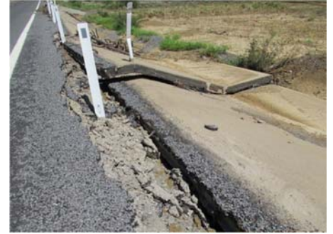
Flinders Highway – erosion behind concrete batters from Gulf of Carpentaria Monsoon Trough (December 2015–January 2016)
