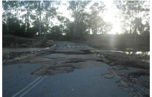
Damage to Callide Creek culvert crossing on Linkes Road after Tropical Cyclone Oswald
