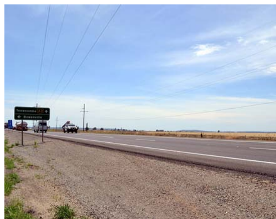
Completed works on Warrego Highway—Bowenville section
