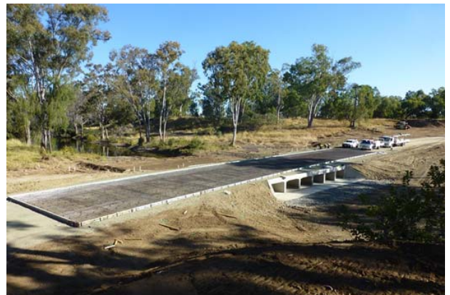
Above: Reconstruction and betterment works underway
