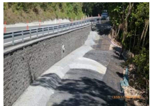
Yarrabah Range Road betterment project following completion—September 2014
