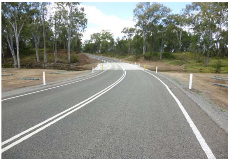
Callide Creek culvert crossing on Linkes Road betterment project after completion
