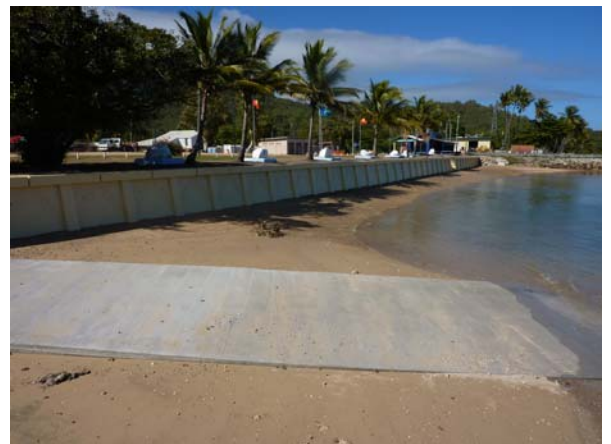
The completed Palm Island seawall reconstruction project - July 2014
