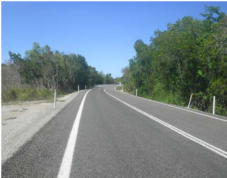
Works completed on Ingham–Halifax–Bemerside Road in December 2014
