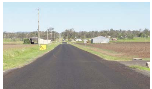
Above: Works nearing completion—November 2013
