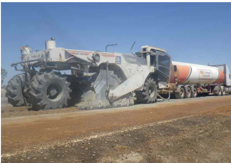
Above: in-situ pavement stabilization, Landsborough Highway (Winton to Kynuna) - October 2013
