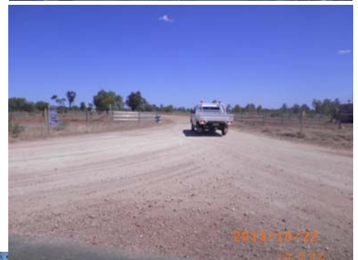
Above: Following completion of works to sections of Portwine Road
