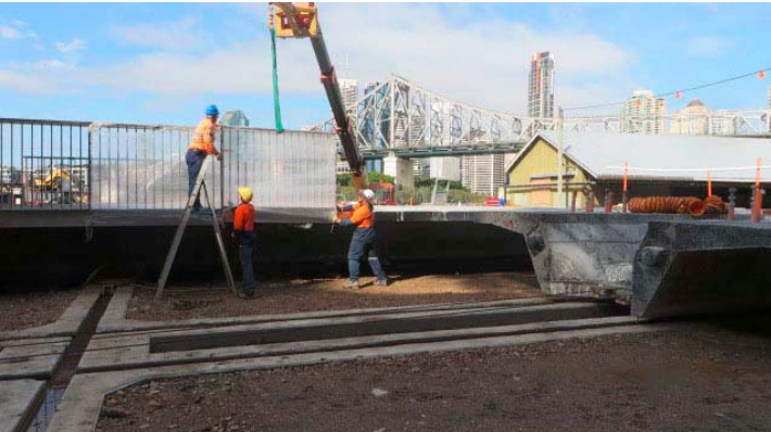
Above: View from the end of the Howard Smith Wharves site (top); balustrade being installed on the pre-cast girders stored on the site (bottom left); and work underway on the northern abutment at the Howard Smith Wharves end (bottom right)
