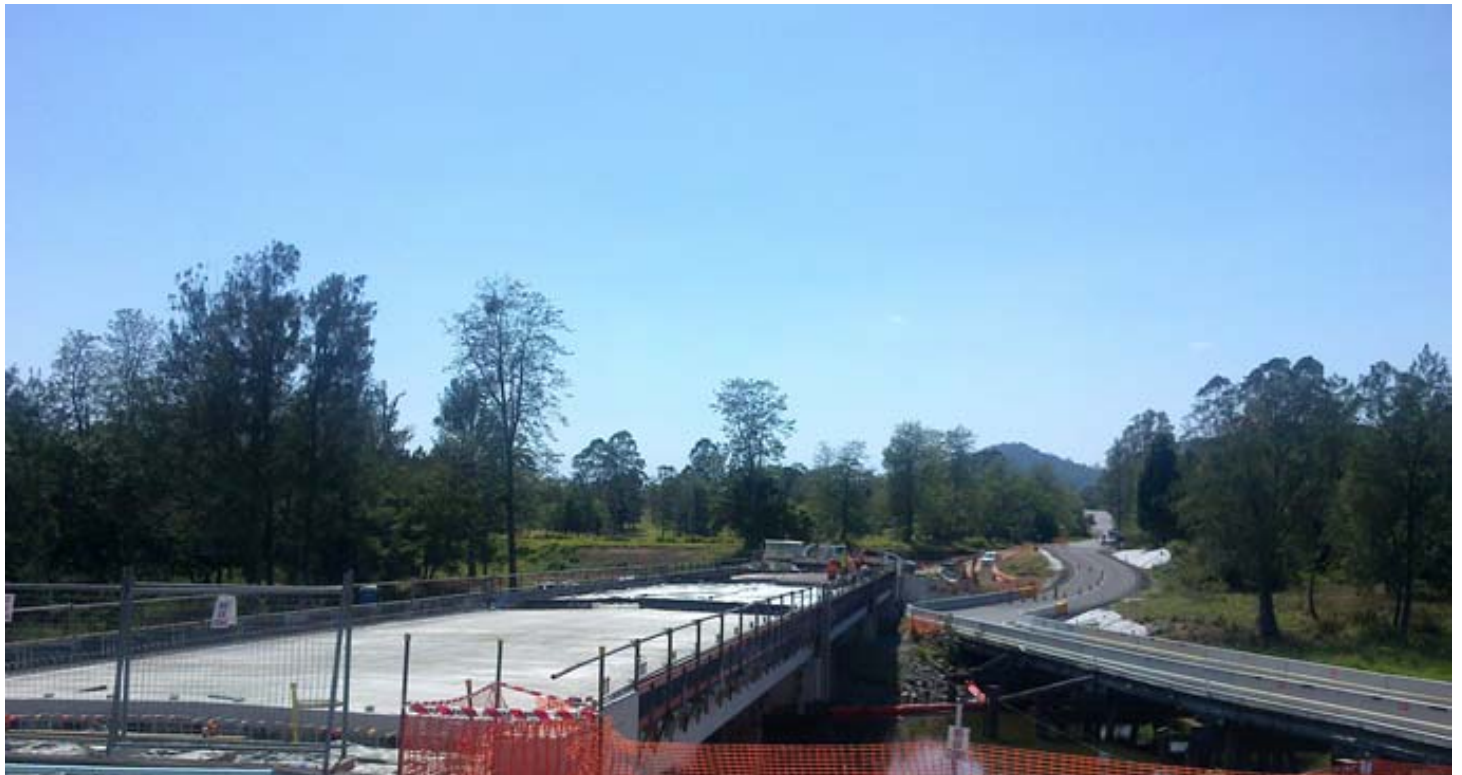
Above: Grigor Bridge new concrete deck, November 2013
