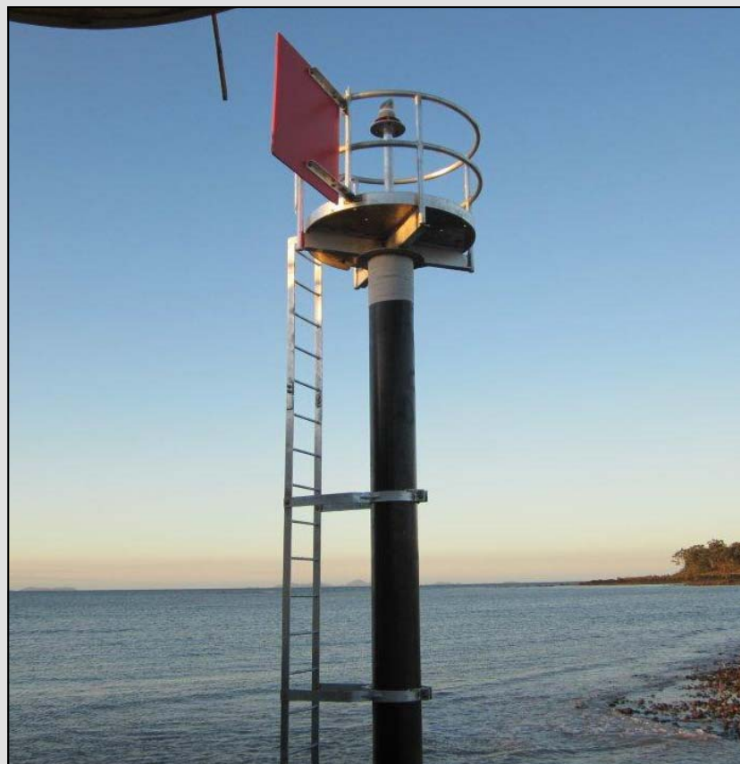
Above: New beacon design in place for Seaforth Creek No 2 Beacon
