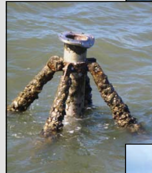
Photos: Typical examples of beacons damaged or destroyed in waters around Mackay and the Whitsundays in 2010.
