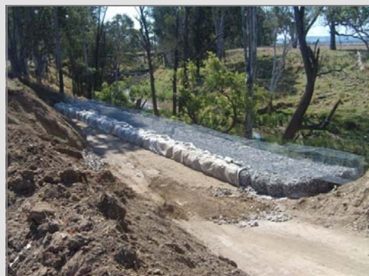
Rock gabion walls are currently being constructed to hold the road in place
