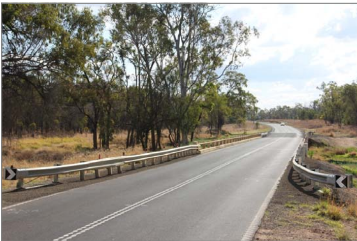
Above: Warrego Highway at Blyth Creek after reconstruction works, August 2012
