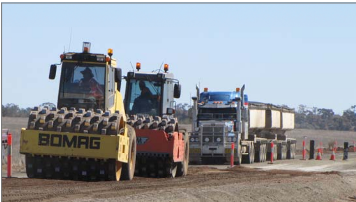
Above: Landsborough Highway near Morven – during construction
