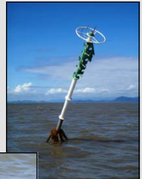
Photos: Typical examples of beacons damaged or destroyed in waters around Mackay and the Whitsundays in 2010.
