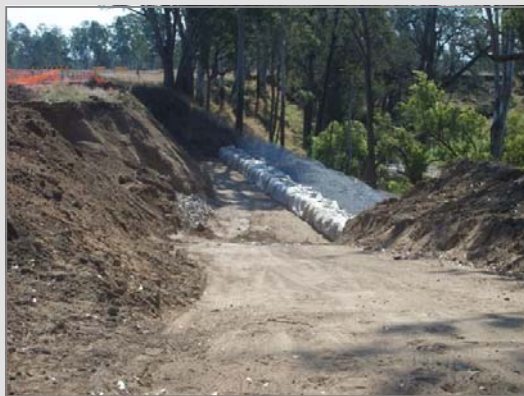
Rock gabion walls are currently being constructed to hold the road in place
