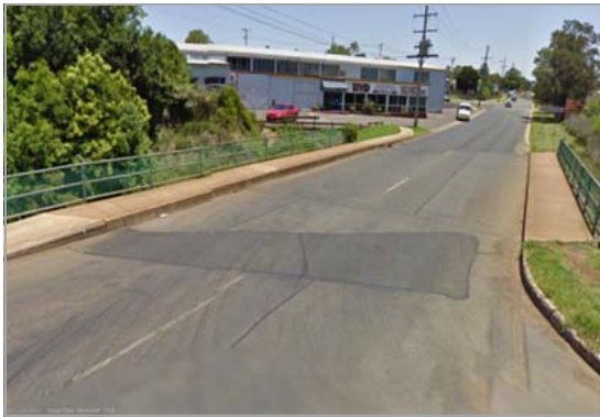
Pre-January 2011 site condition
