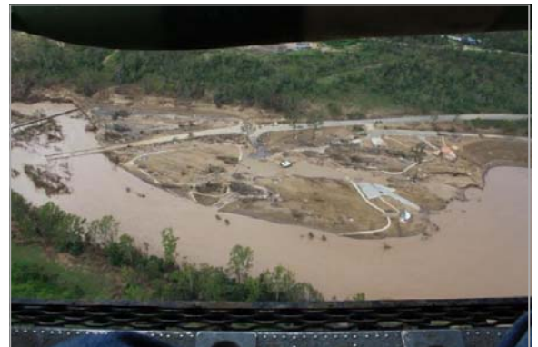
Above: Aerial view of damage to Colleges Crossing Recreation Reserve
