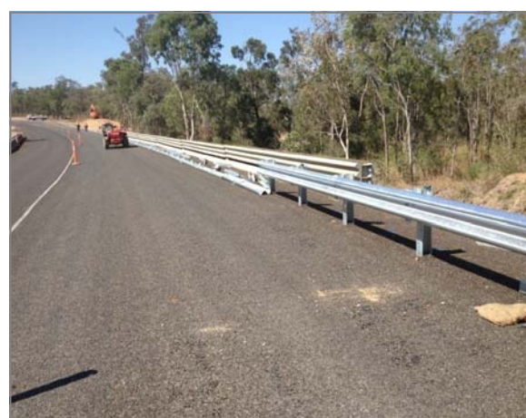
Above: Installing the guardrail on the Peak Downs Highway.
