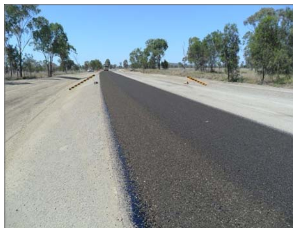
Above: Sealing works on the Suttor Developmental Road.
