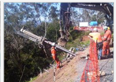
Above: Soil nailing underway to repair the road at Cunninghams Gap
