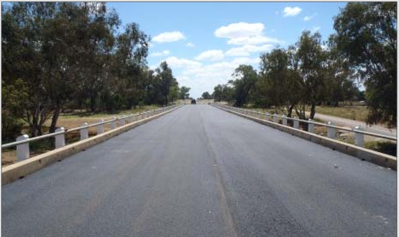
Above: October 2012 - Newly completed resurfacing (Barcoo River Bridge, Landsborough Highway)
