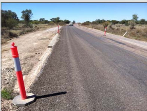
Above: During reconstruction works - following first seal at Rutchillo Creek Floodway
