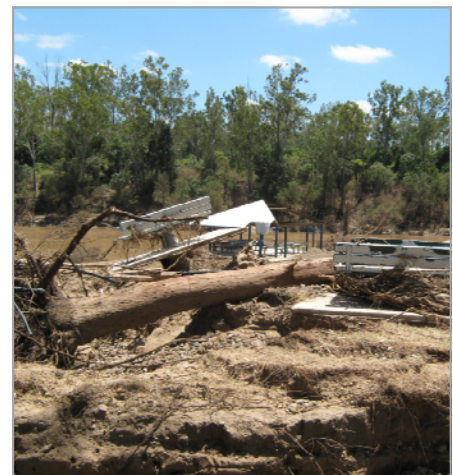
Above: Before - damage to Colleges Crossing Reserve
