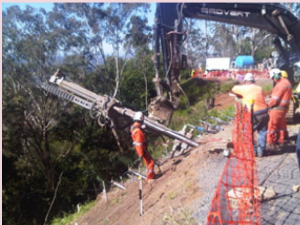
Soil nailing underway to repair the Toowoomba Range road network
