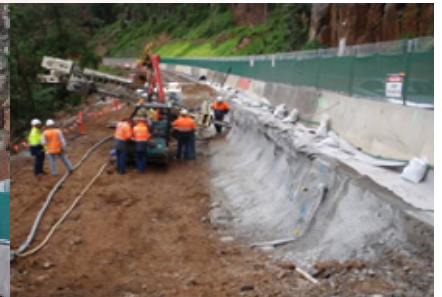
Progress continues at the Cunningham's Gap site
