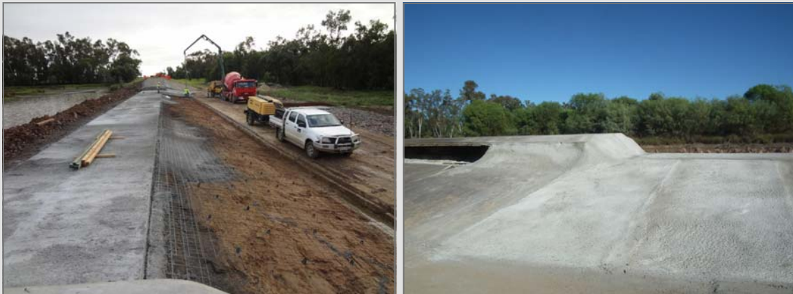
Above left: Moolabah Weir under repair
