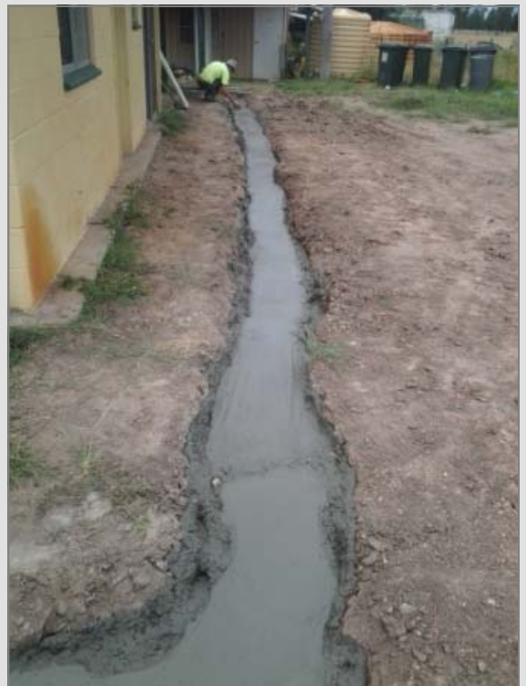
Above: Builders completing repairs to septic tank.
