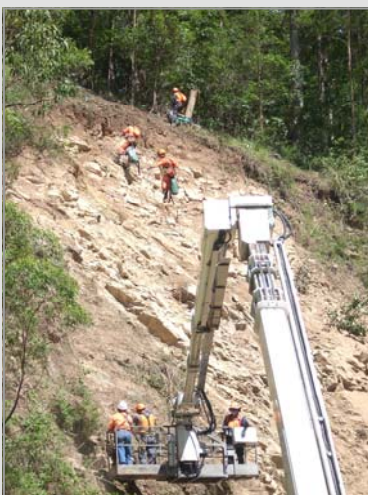
Above: Descaling crews at Hairpin Bend site during emergent works.
